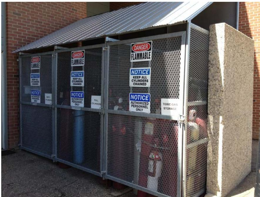
**Figure 10: Outdoor cylinder storage facility. Image courtesy of Safety Resources.**
